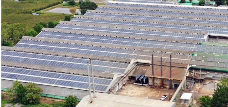
The Prachuab Fruit Canning Co., Ltd. (Praff) Prachuab khiri khan Capacity : 507.28 kWp Solar Rooftop
